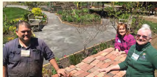
May 11: Red brick pavers are stacked (over several days) near the work area, by Garden Crew volunteers. Karl, Karen, and Mary are photographed.
